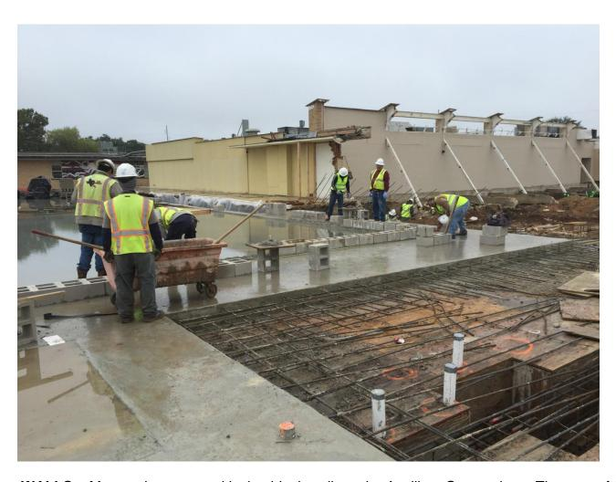
**WALLS** – Masons have started laying block walls at the Auxiliary Gymnasium. The start of the masonry work is on schedule.
