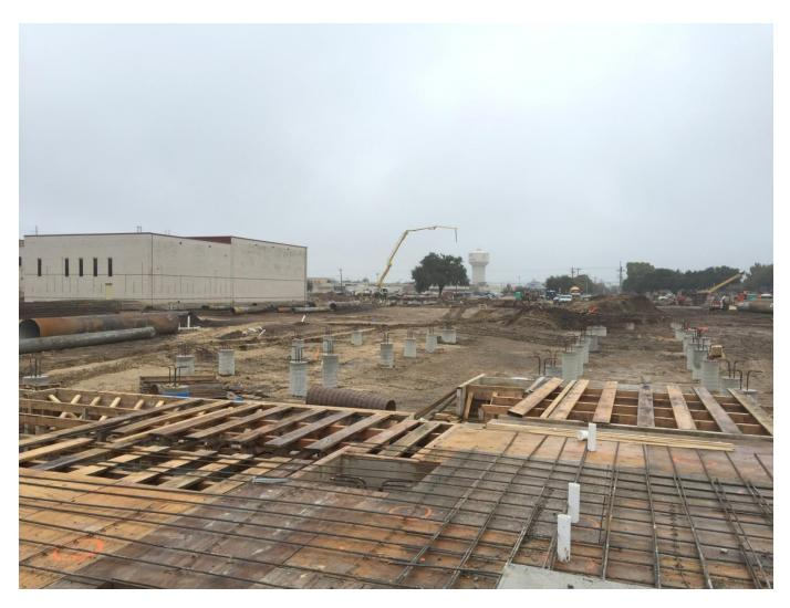
**FOUNDATION** – Foundation Formwork installation is in progress. No pier drilling on this day due to muddy site conditions.
