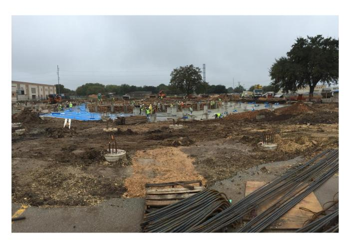
**FOUNDATION** – Under floor concrete mud slab and moisture protection installation is in progress at the Performing Arts Center (PAC). The PAC is located at the former ROTC Building site.
